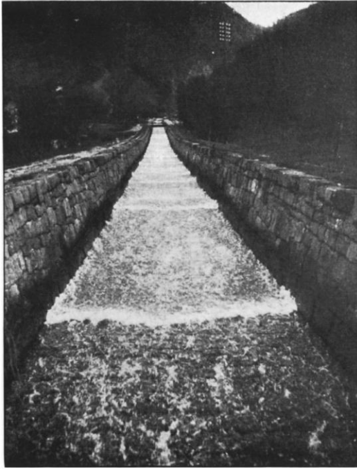
FIG. 1.—ROLL-WAVES IN THE GRÜNNBACH CONDUIT.
