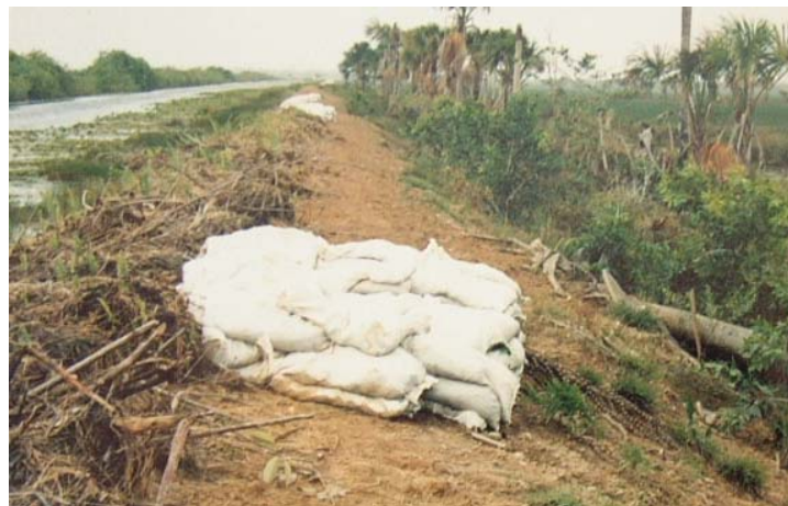
Photo 12: EDWC East Dam temporary crest repairs using vegetation
