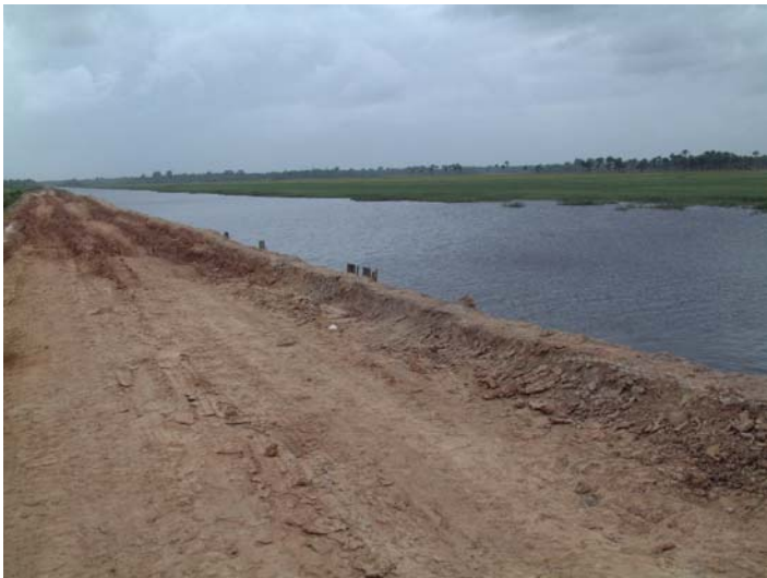
Photo 18: Boersarie South East Dam typical section
