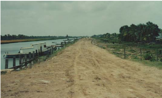
Photo 15: Boersarie East Dam typical view
