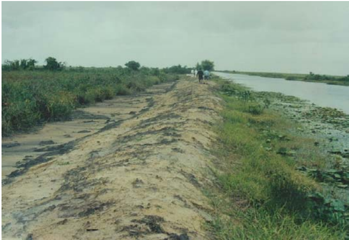
Photo 3: EDWC North Dam
