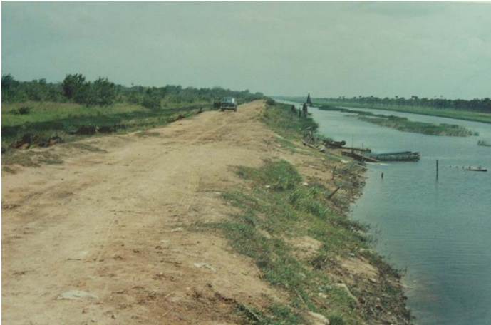
Photo 16: Boersarie East Dam typical view
