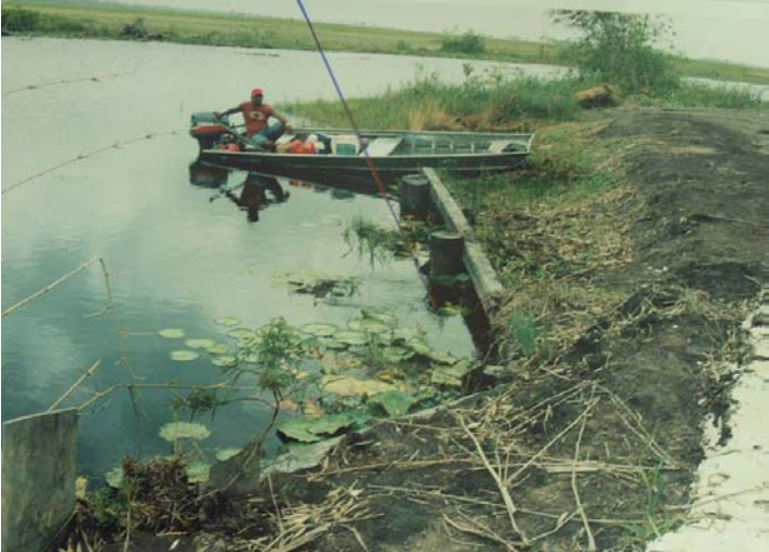
Photo 14: EDWC North East Dam leak at Enmore Koker
