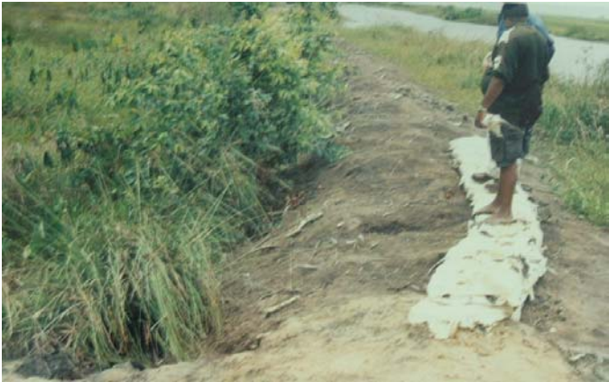
Photo 2: EDWC North Dam
