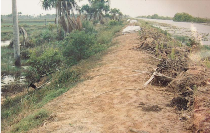
Photo 13: EDWC East Dam temporary crest repairs using vegetation
