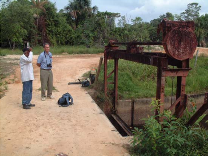
Photo 19: Boersarie Patosi Relief Sluice
