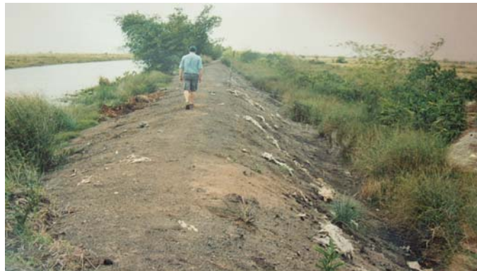
Photo 8: EDWC North East Dam crest reinstatement: Repairs to crest
