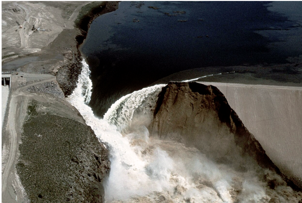
Fig. 4 Failure of Teton Dam, on the Teton river, in eastern Idaho, on June 5, 1976, possibly a rare instance of a mixed kinematic-dynamic wave.
