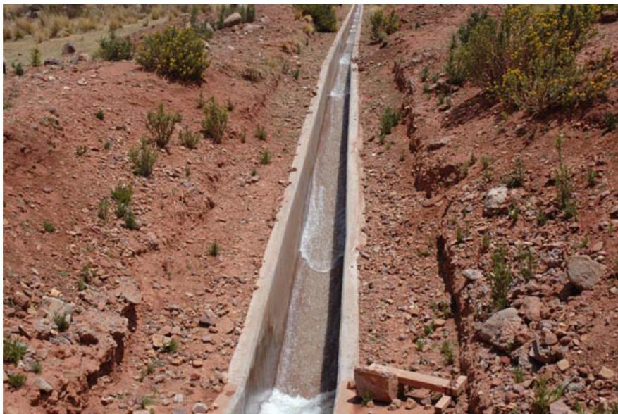
Fig. 2 A train of roll waves in a lateral canal, Cabana-Mañazo irrigation, Puno, Peru.
