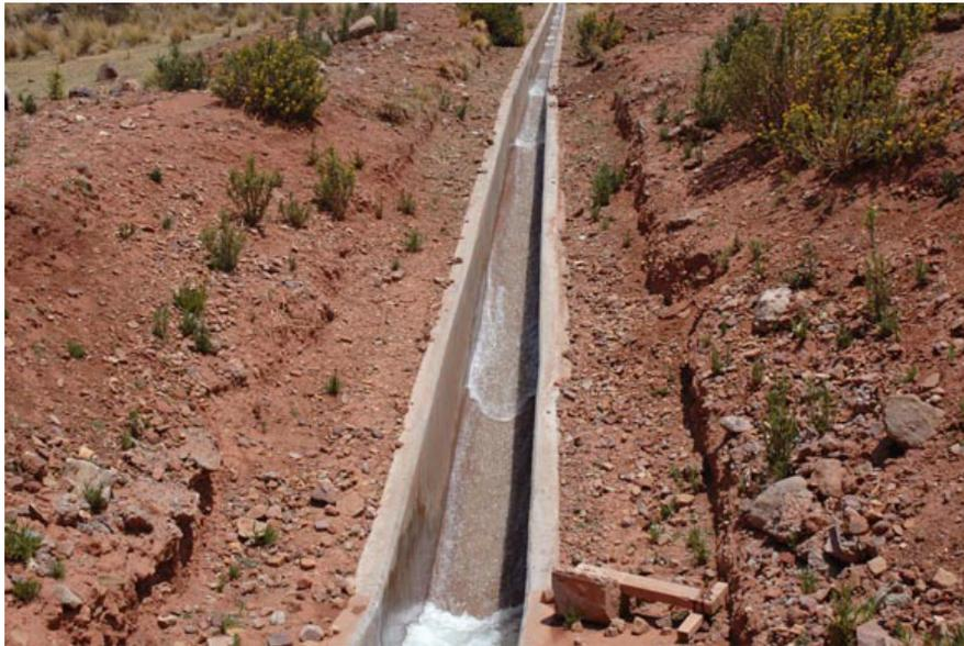
Fig. 2 Roll waves in a steep lateral canal, Cabana-Mañazo irrigation, Puno, Peru.
