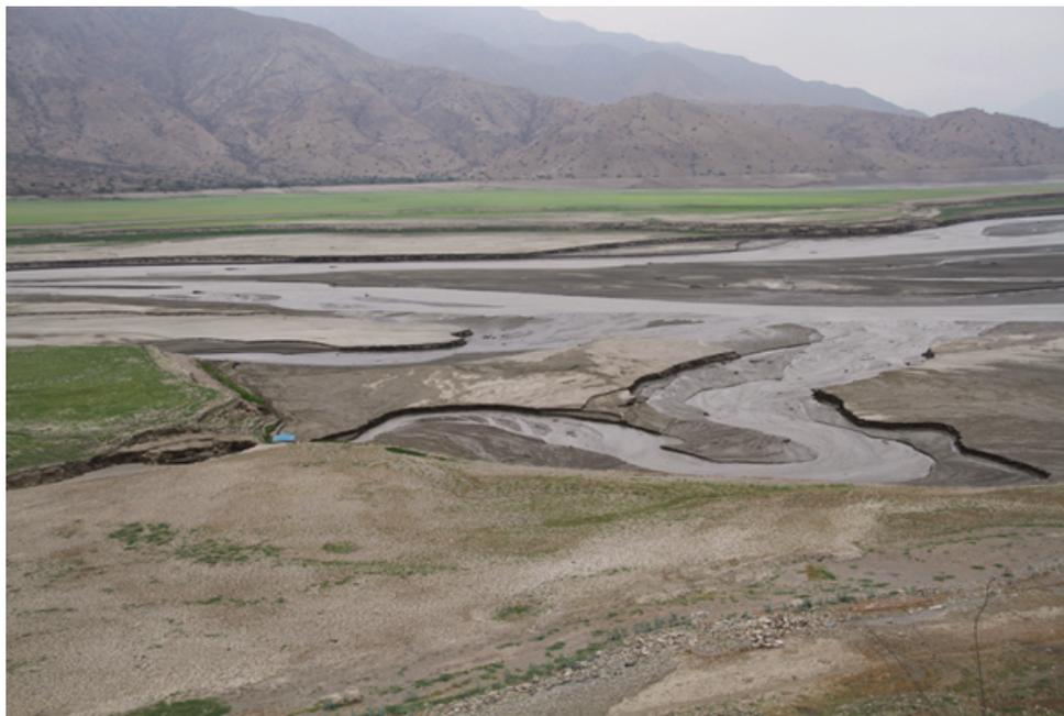
Fig. 1 Sedimentation at Gallito Ciego reservoir, La Libertad, Peru.
